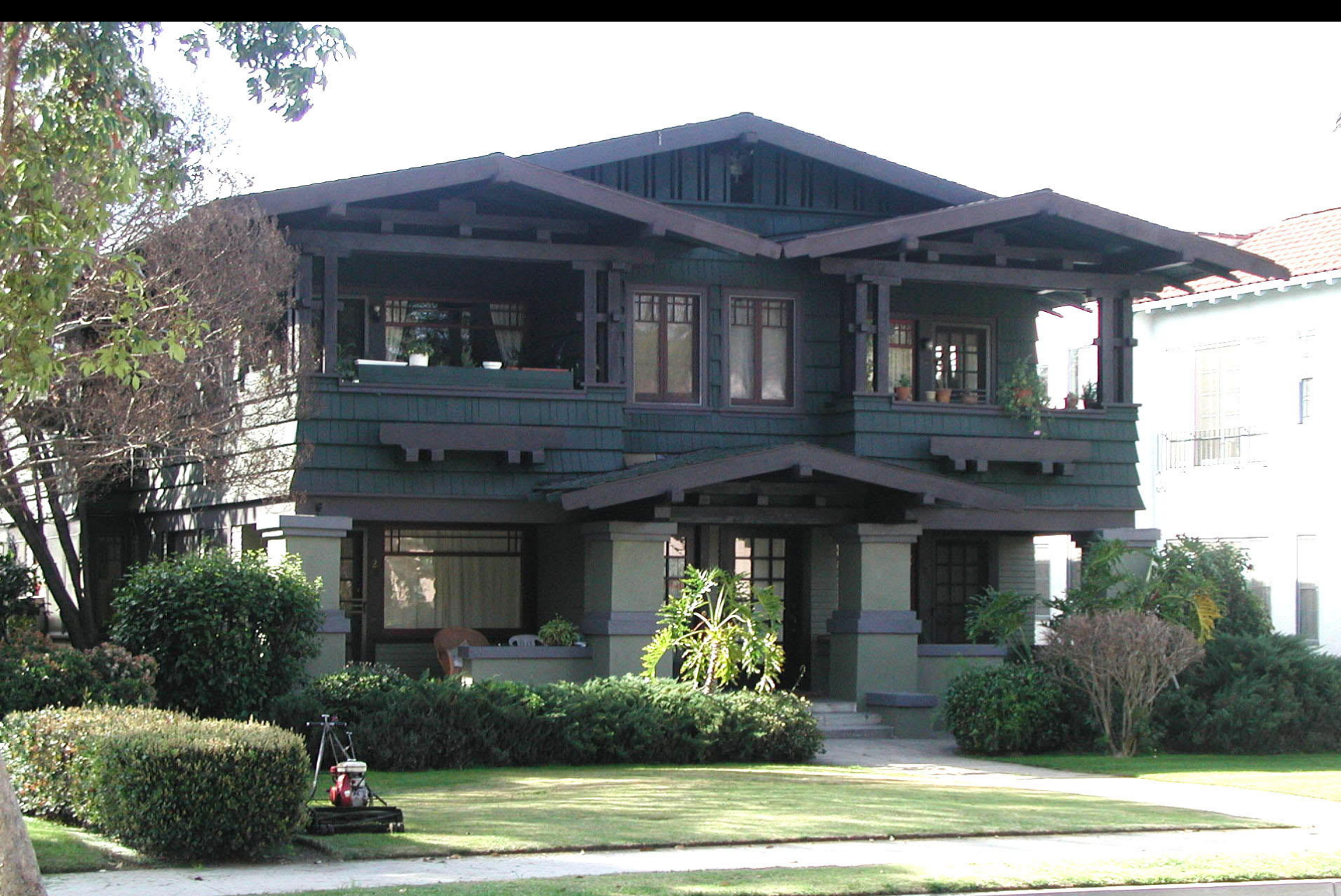
Shared House (Quadplex)
