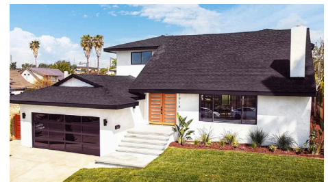
Before (top) and after (bottom) image of 1914 W. Victoria Ave. An example of a property brought into compliance through code enforcement actions.
