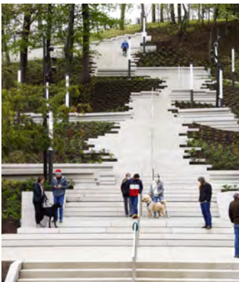
4 Stairs, ramps, and public art in the Sculpture Park leading to the Rio Hondo Channel.
