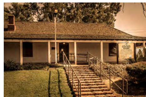
The Sanchez Adobe is the oldest known built resource in Montebello, and is a rare example of an extant structure associated with Southern California’s Mexican-era roots.
