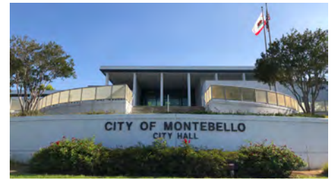
Designed by architect William Allen, the new City Hall was designed in the Mid-Century Modern style and stood as a bold testament to the city’s remarkable growth in the postwar period. Allen also designed a new public library and police station within the civic center complex, both of which were erected in 1964.
