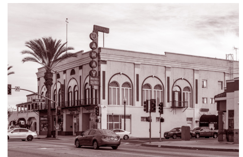
In 1927, a large new fraternal lodge operated by the Independent Order of Odd Fellows opened at the corner of Whittier Boulevard and 10 th Street (the building is currently used as a dance hall).
