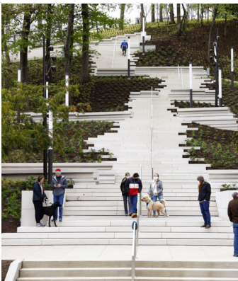
4 Stairs, ramps, and public art in the Sculpture Park leading to the Rio Hondo Channel.
